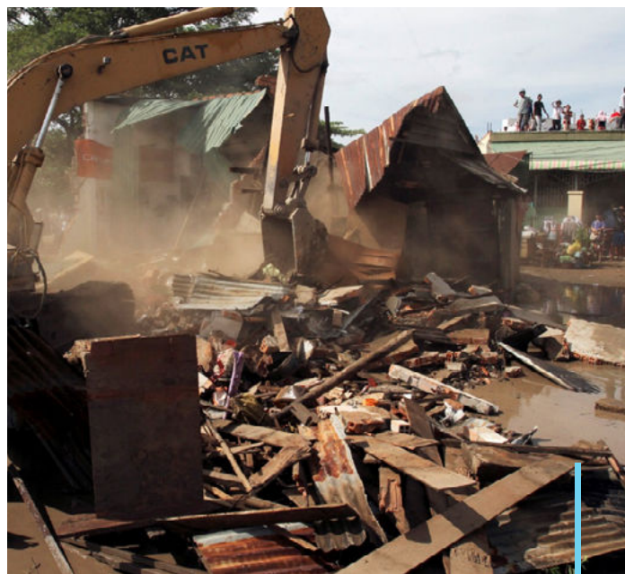
Demolition of Boeung Kak Lake community.
