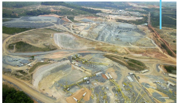
Belo Monte Dam construction 2013.
